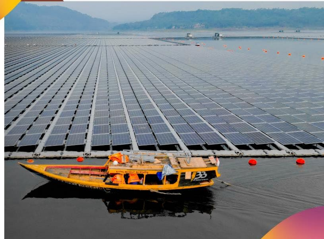
Cirata Floating Solar Power Plant, 192 MWp
