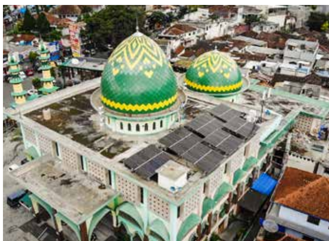
Solar panels installation with up to 20 kWp capacity at An-Nuur Mosque rooftop located in Batu City, East Java, Indonesia.
