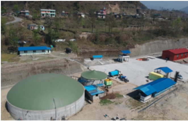
A municipal waste-based biogas plant is installed the capacity of 4,200 m 3 in Pokhara City, Gandaki Province, Nepal
